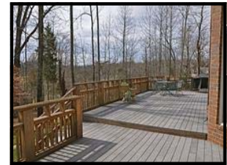
Back deck extends the full length of the home
